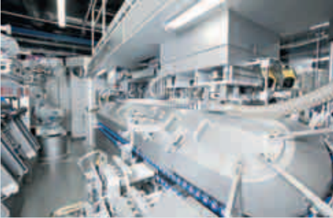
Overall view of the TFS 80-8 with the internal machine transport system in the foreground.
