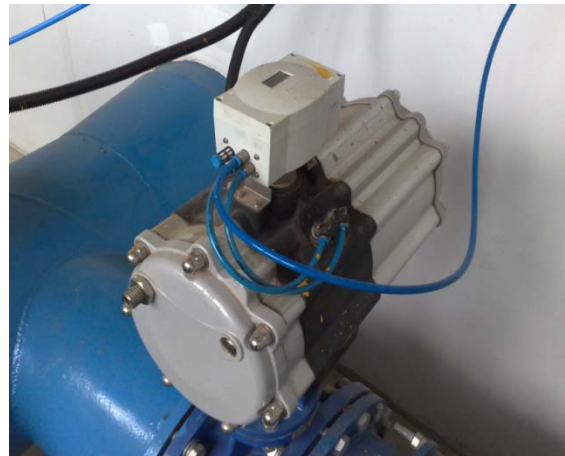
Figure 11: Control valve.
