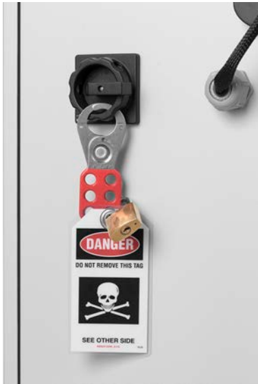
Figure 11. Installation of a lockout hasp, padlock, and tag.
