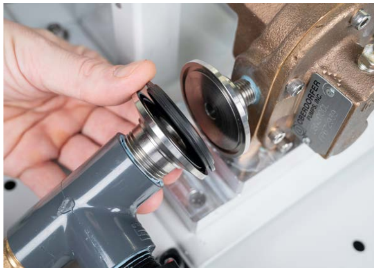
Figure 45: Pressing the fittings together, with the gasket in-between.
