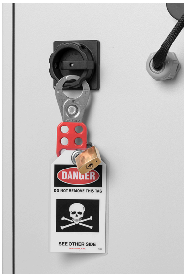
Figure 9. Installation of a lockout hasp, padlock, and tag.
