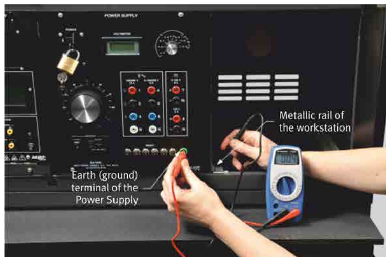
Figure 33: Verifying the earth (ground) terminal connection of the Power Supply with an ohmmeter.
