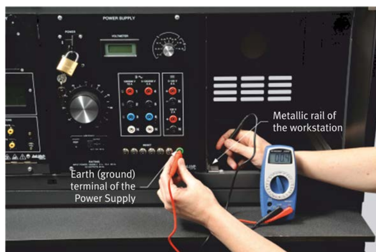
Figure 32: Verifying the earth (ground) terminal connection of the Power Supply with an ohmmeter.
