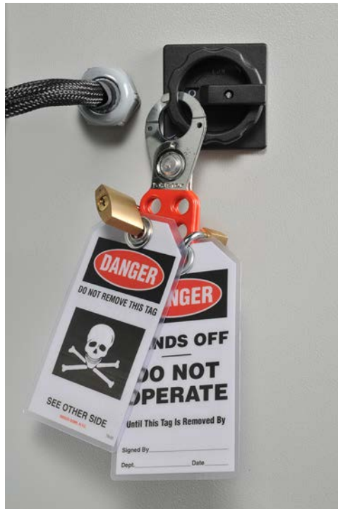
Figure 38: Installation of the lockout hasp, padlocks and tags.
