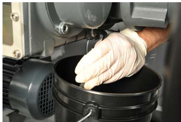
Figure 56: Removing the drain plug.
