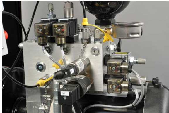
Figure 23: Hot hydraulic unit solenoids.
