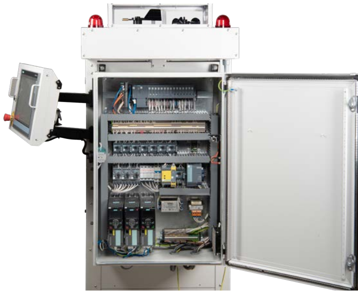
Figure 30: Electrical panel.
