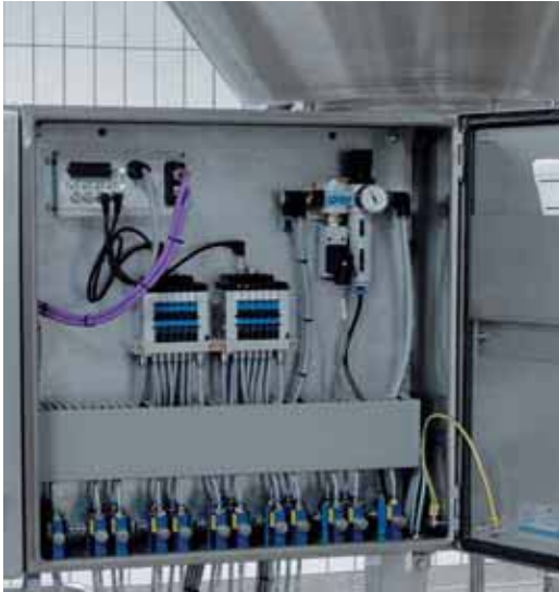
Breweries are classic hybrid industries: Process automation with CPV fieldbus valve terminals on the brewing floor.
