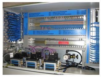
Figure 14: Valve terminal cabinet in ATEX zone 2 with valves for a safety instrumented system.
