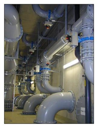
Figure 8: Pipe gallery in a water treatment system
