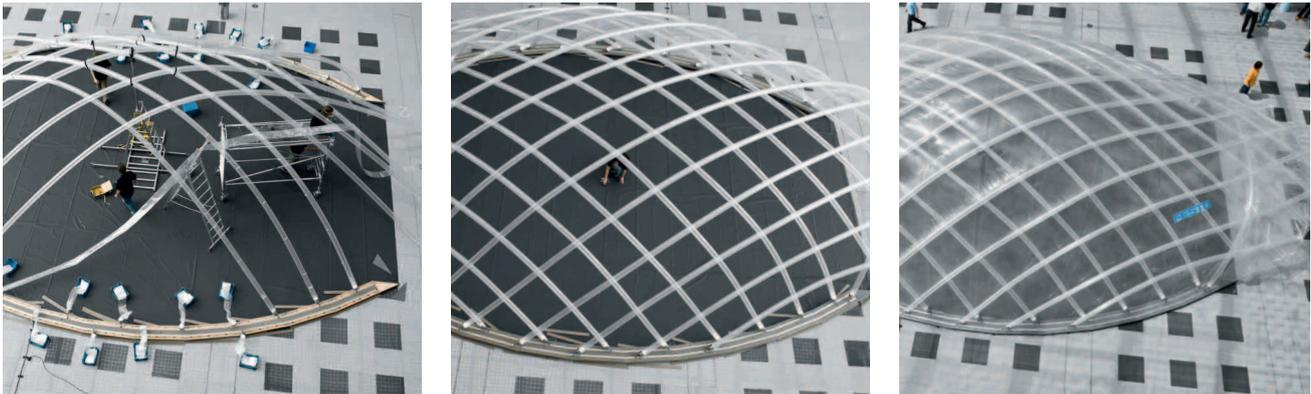
Self-righting tubes: fast assembly time without time-intensive auxiliary constructions
