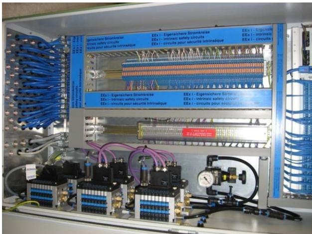
Figure 14: Valve terminal cabinet in ATEX zone 2 with valves for a safety instrumented system.
