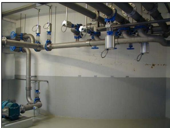
Figure 9: Pipe gallery in a wastewater treatment plant
