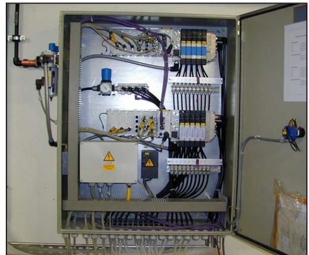
Figure 10: Control cabinet with valve terminal
