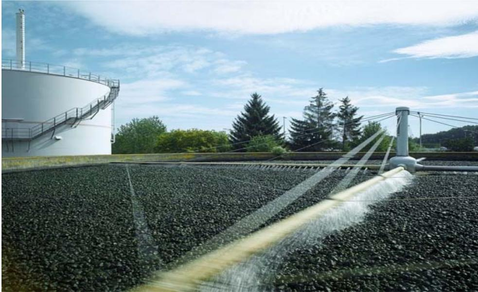
Figure 4: Trickling filter system.
