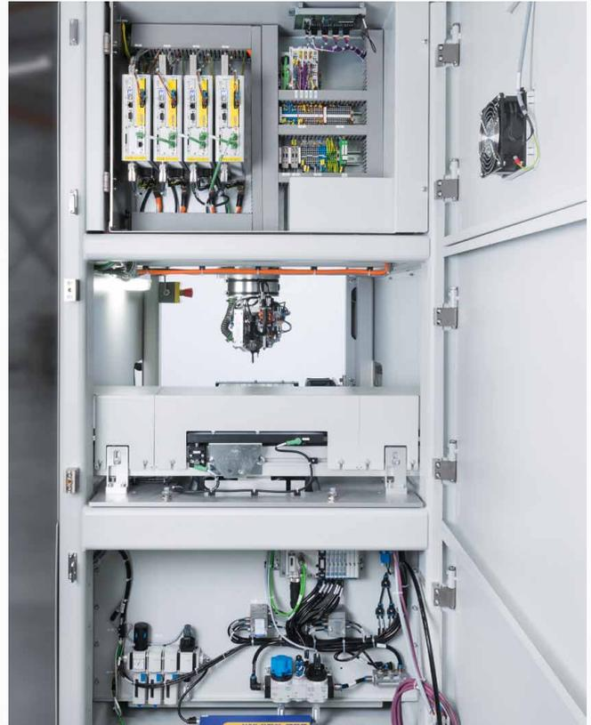
**All in one:** mechanical components, servo motors, controllers, compressed air preparation and valve terminals from Festo.
