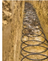
Ground loop installation
