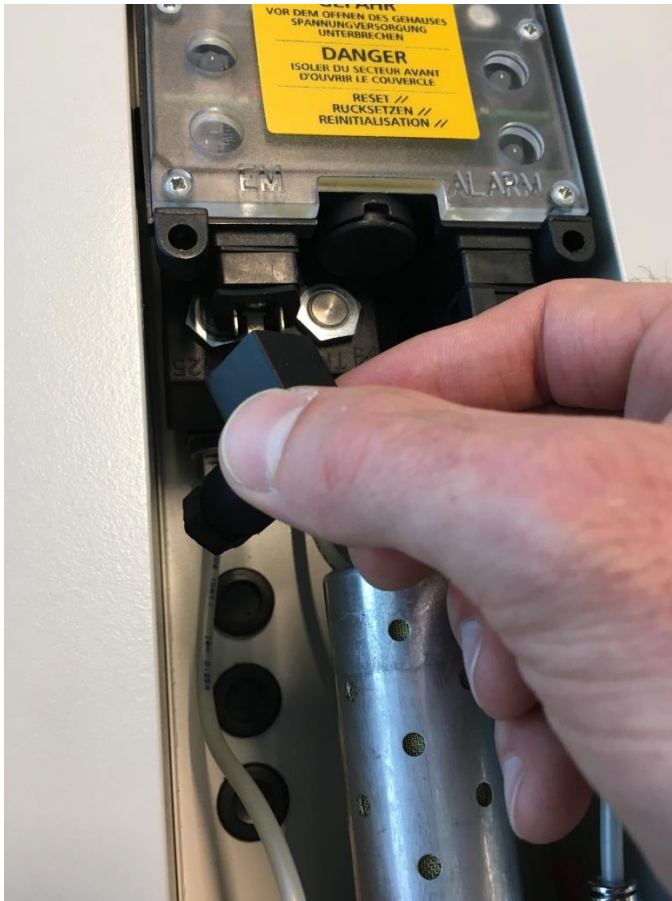
Figure 7: PDAD default status – DIN plug with pre-set jumper connected to EM contact
