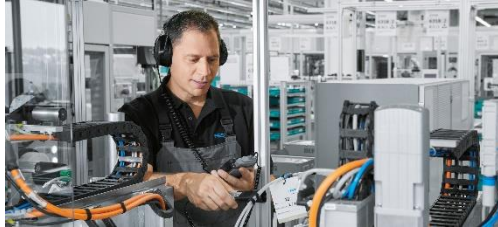
Energy Saving Services
