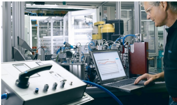
Figure 10: Measurement of compressed air consumption
