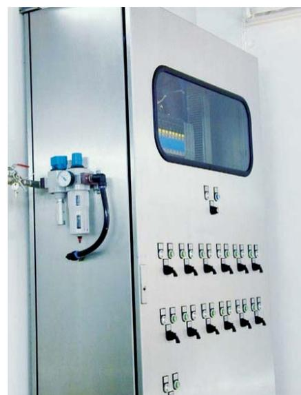
**Fig. 4:** Valve terminal in control cabinet with convenient manual control panel
