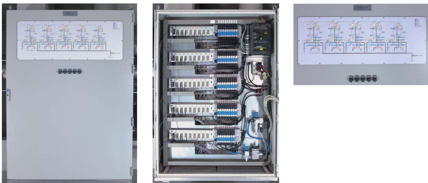
Fig. 5: Valve terminal in control cabinet with schematic plant diagram
