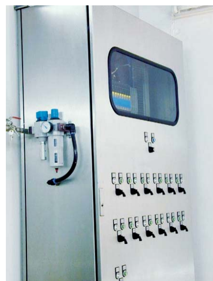
Fig. 4: Valve terminal in control cabinet with convenient manual control panel
